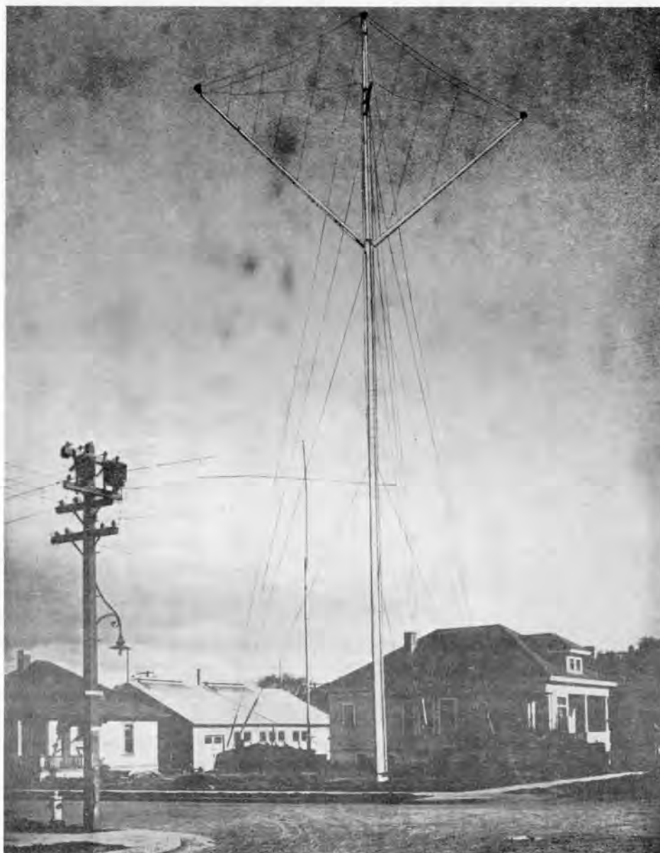
Federal's first laboratory and factory located on Emerson Street and Channing Avenue, Palo Alto, California. The first Federal arcs were manufactured in the corrugated iron shed behind the cottage, which was used as a laboratory. The shed became a place of historical significance when, in 1912, Dr. Lee de Forest and his assistants developed the audion amplifier and vacuum tube oscillator there.
